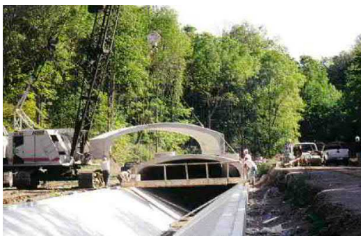
Figure 4.1 – CSO Facility Under Construction (RVA Photo)
